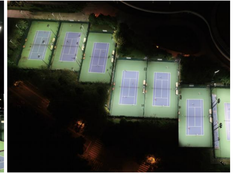
Guangdong Olympic Center Tennis Court
